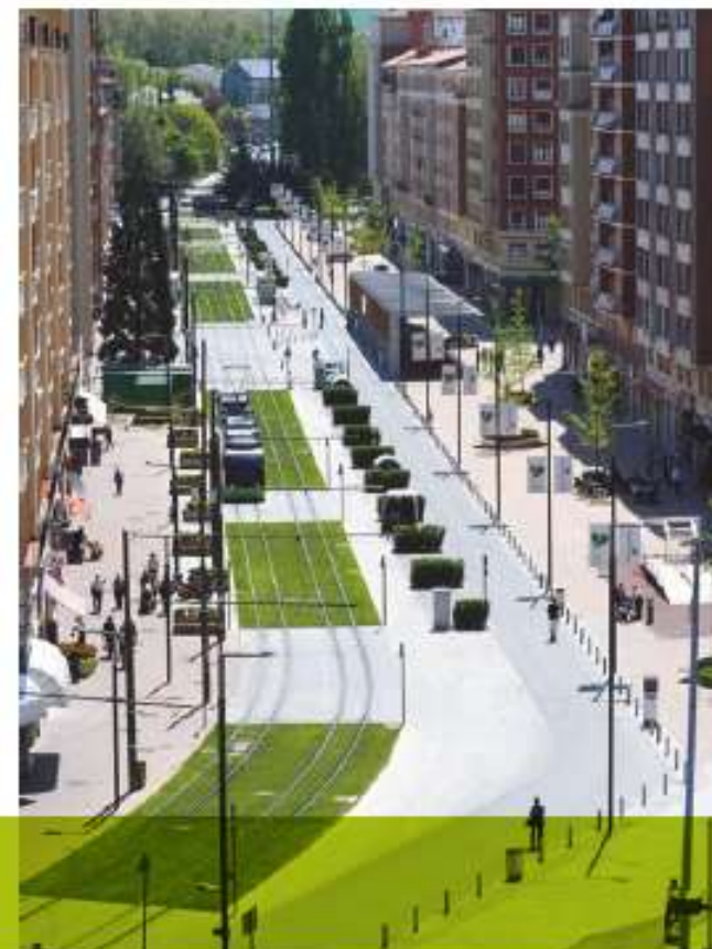
▼ Transformation of Sancho el Sablo street, after the implementation of the first superblock in Vitoria-Gasteiz.
